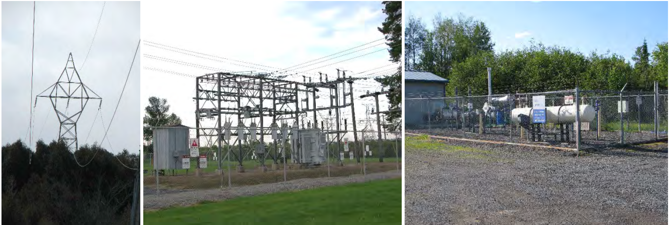
Powerline rights-of-way, power facilities and pipelines are kept clear of vegetation for safety.
